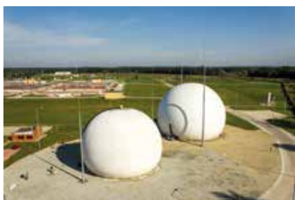
/ Balony na biogaz
